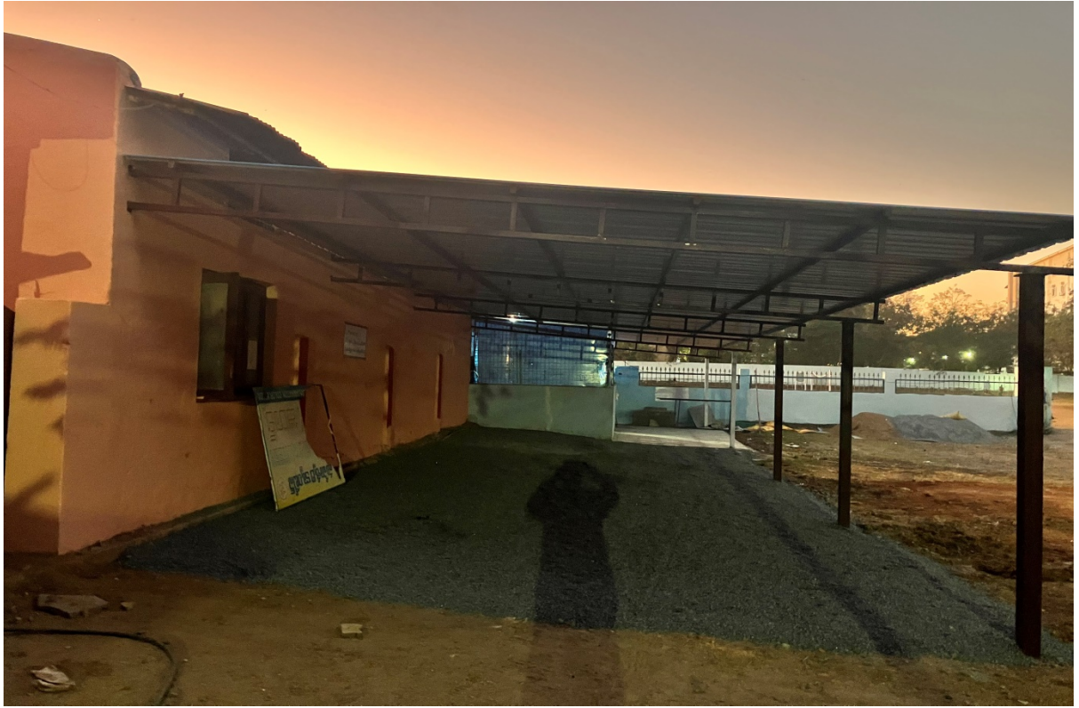
Newly constructed vehicle shed came into use w.e.f 1-1-2023
