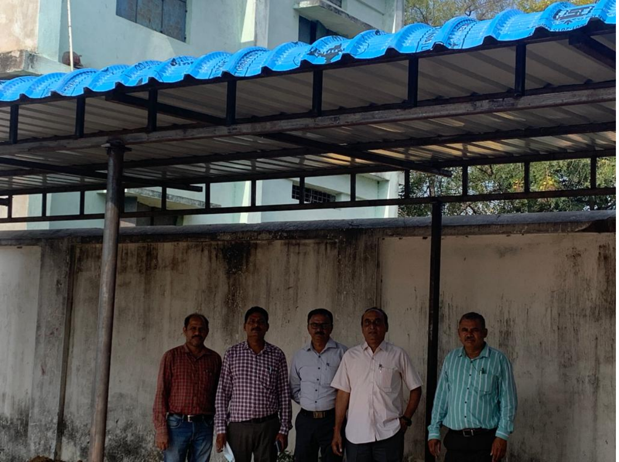
Front view of Newly Built Vehicle Shed with Alumni Funds and came into use w.e.f. 8-8-2022
